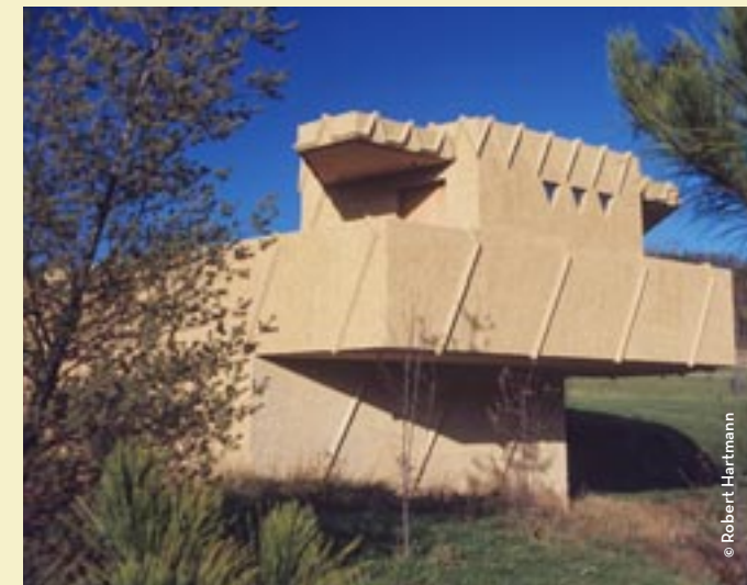
The Gatehouse as it appeared during construction in 1968, top, and shortly after its completion the following year, above
